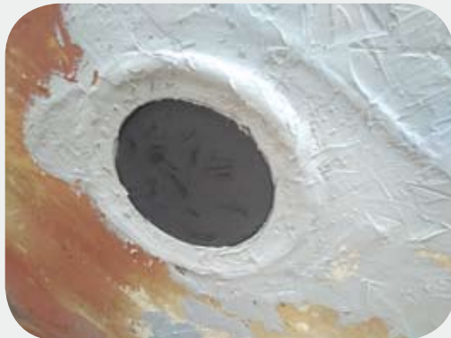
New anode installed
