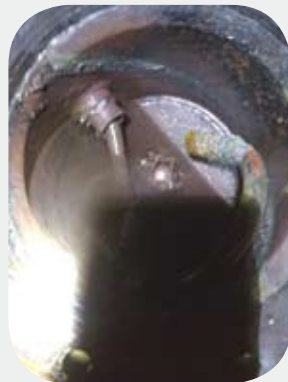
Anode leakage
