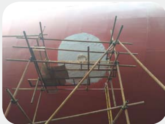
Di-electric shield applied
