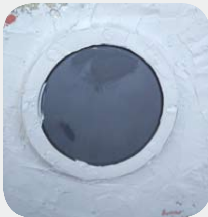
New anode installed
